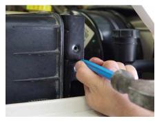
37. Mark the location of where your hole needs to be drilled using a center punch.
